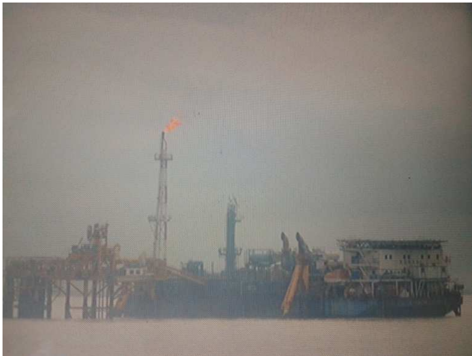
An oil platform on the high sea. Picture taken while waiting for the Nigerian navy to escort us
